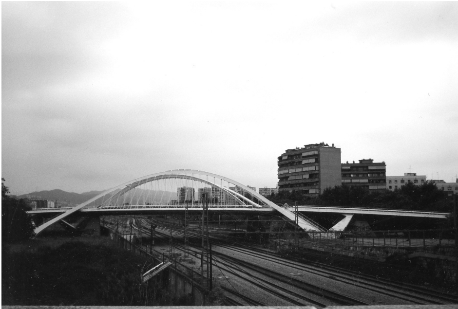
Figure 6] Santiago Calatrava's Bridge in Barcelona (photo by author).
