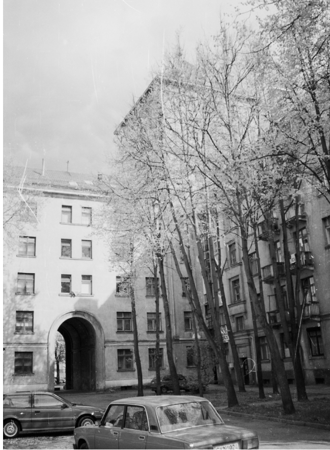
Figure 1] Pergalė factory residential buildings, Kaunas. Arch. Jokūbas Peras, 1956 (photo by author, 2001).
