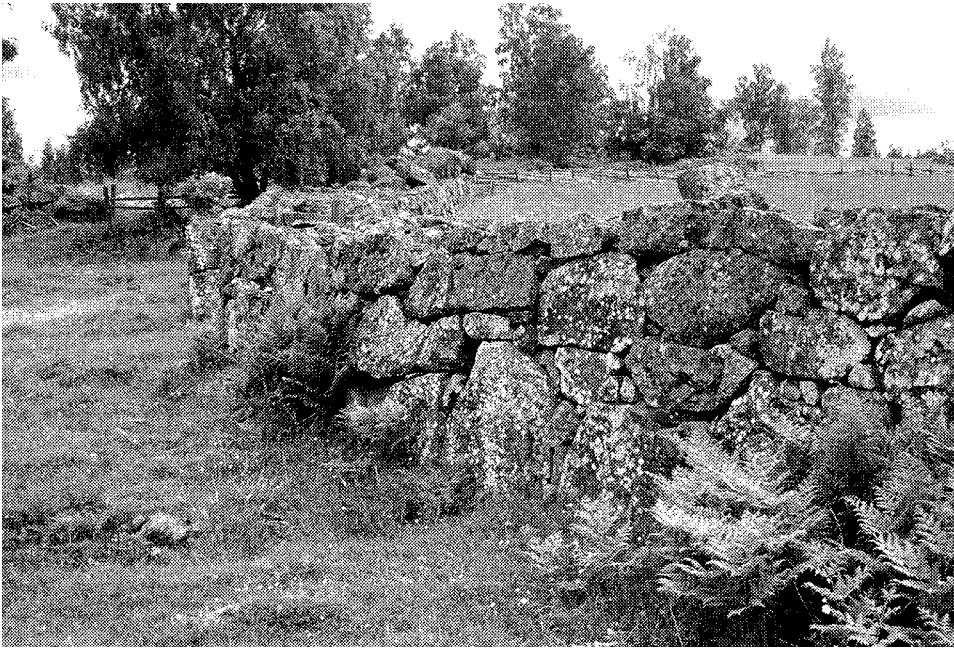
Figure 3. Traditional stone fence in Bråbygden in 1997 (photo by author).
